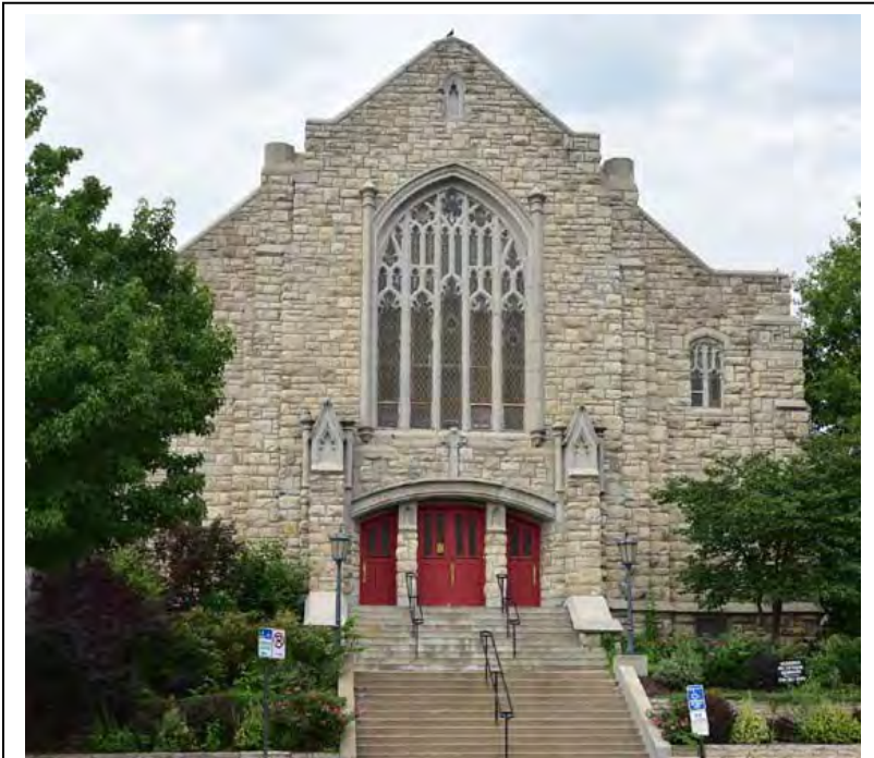
Figure 82. First Swedish Baptist Church, 3931 Washington Street
