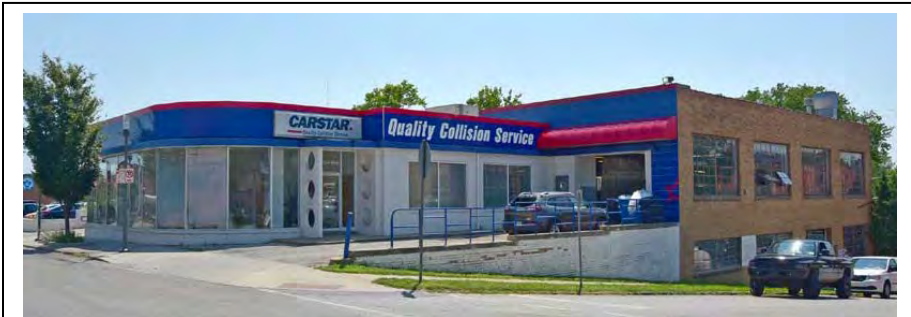
Figure 86. Automobile Sales and Service Building, 4200 Main Street
